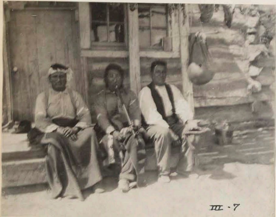
Pannich bucket hanging in place.
