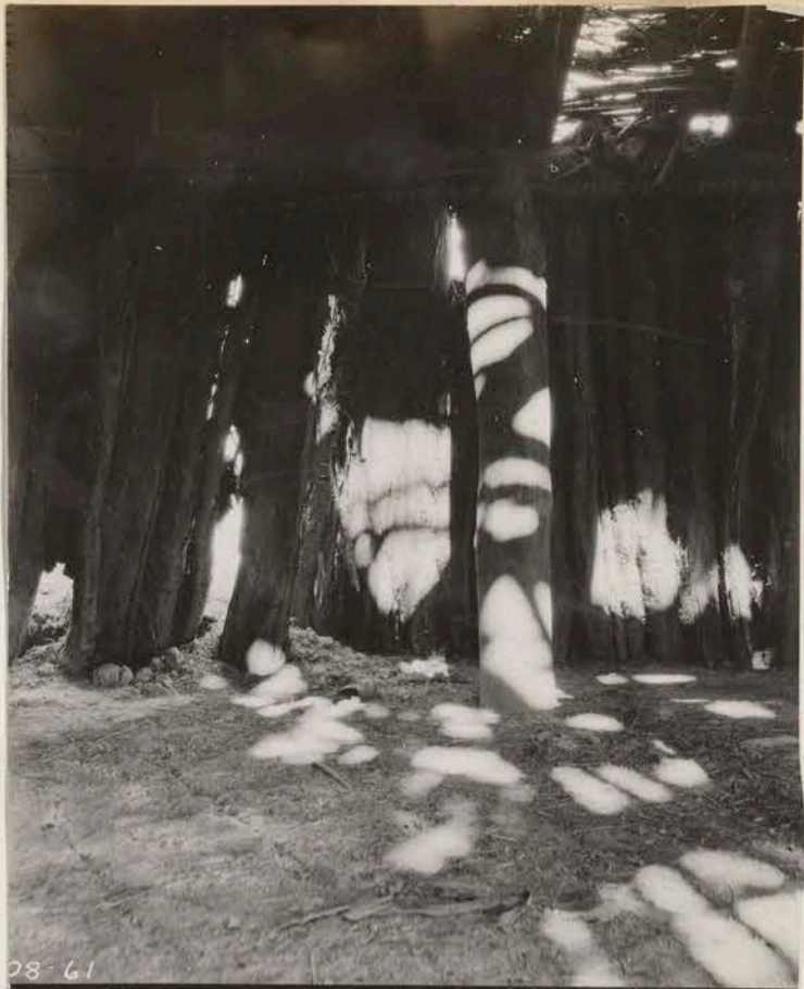
Owl Woman's lodge in 1908 - interior view. Lodge falling into bad condition
