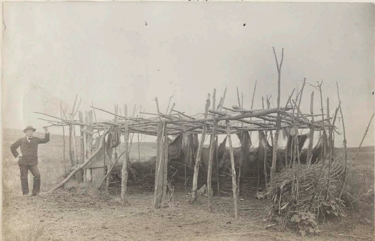
Self by frame of old cabin. Note how walls are built of willows. Ft. Yates 1905
