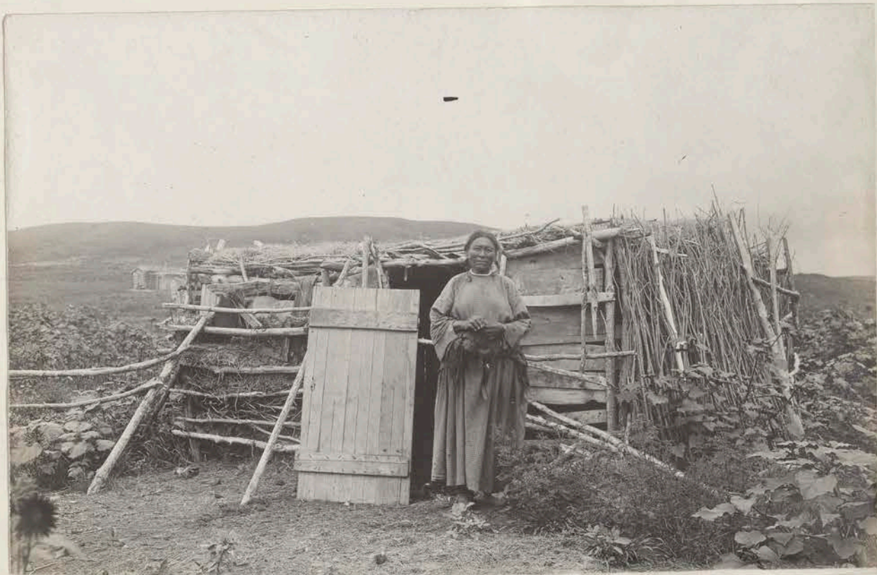
Curious mingling of old and new. Rude sod-cabin, built in part with nails and boards and in part with willows and even with walls stuffed with willows and straw, as see on right. The cabin was used as a barn. Owner stands in front.
