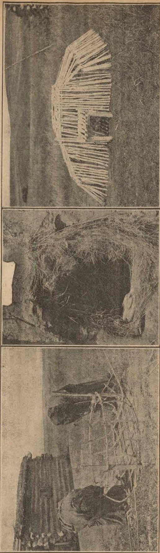
Building Activities in the Hidatsa Villages of Western North Dakota. Left, Bottom Frame of a Bull Boat, Made of "Mahohishah" Willow, to be Covered with Skin. Center, Section of a Cache Pit Made by Buffalo Bird Woman in the Bank of the Missouri to Show How the Indians Stored Their Corn. Right, Model of the Frame of an Earth Lodge—the Large Type Supported by Posts and Beams
